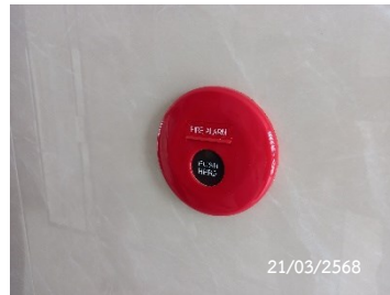
Fire Alarm Manual Station
